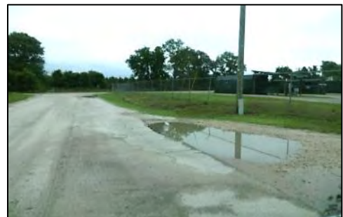
Photograph 6 – Stormwater Ponding
