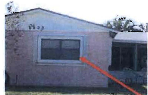
This home was disqualified for a discount because every opening except this window was protected with an impact resistant product.
