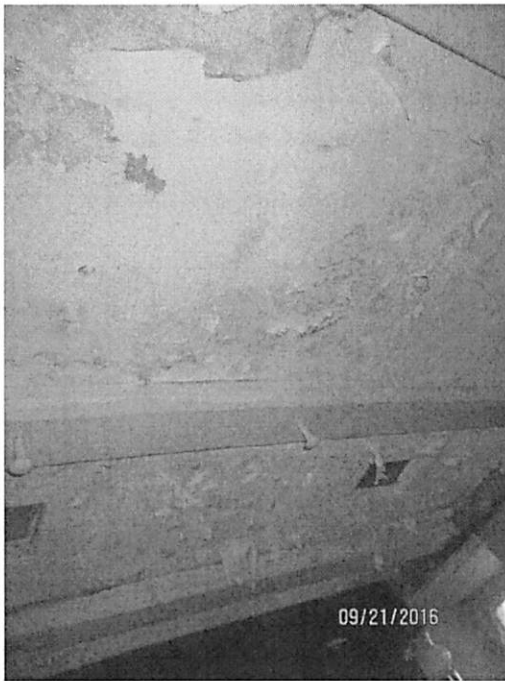
Photo 13. Flaking ceiling paint, aft area.
