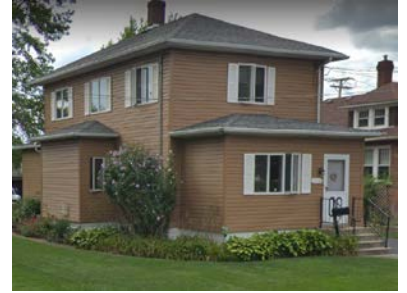
Right: Three houses north (17112) – Vinyl Siding
