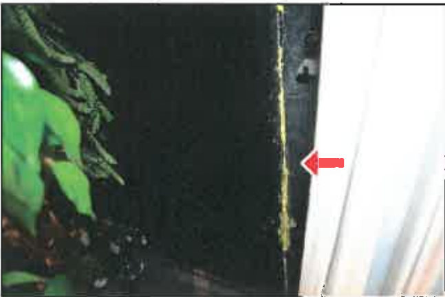
E. Item 14(Picture) Damaged seal at west door
