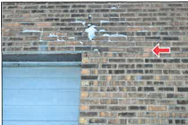
D. Item 6(Picture) Cracks west
