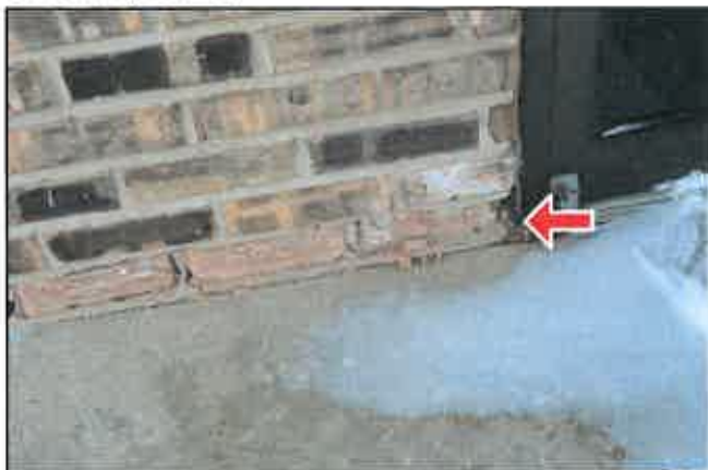
C. Item 2(Picture) Deteriorated bricks at entrance
