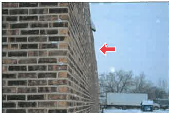
D. Item 2(Picture) West wall damage
