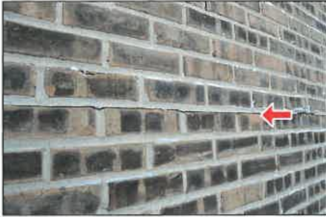
D. Item 1(Picture) Cracked mortar joint
