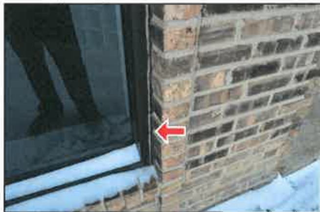
E. Item 4(Picture) Gap at frame
