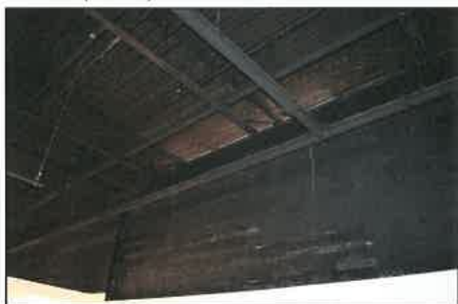
G. Item 3(Picture) Rust at roof deck
