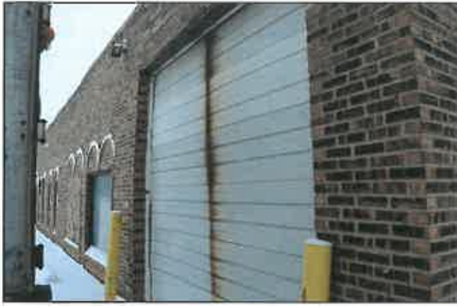
E. Item 7(Picture) Rust at overhead door
