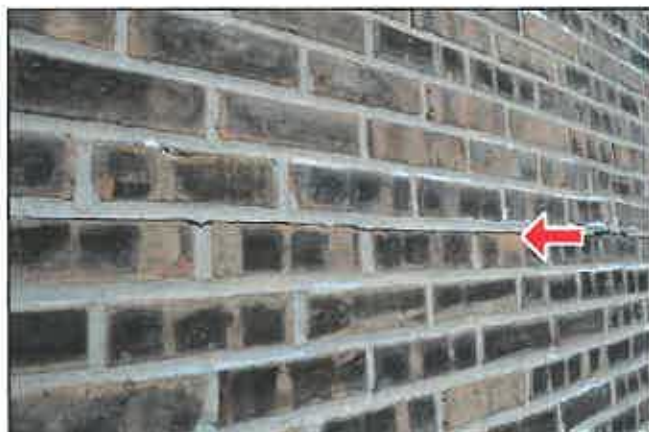
D. Item 1(Picture) Cracked mortar joint
