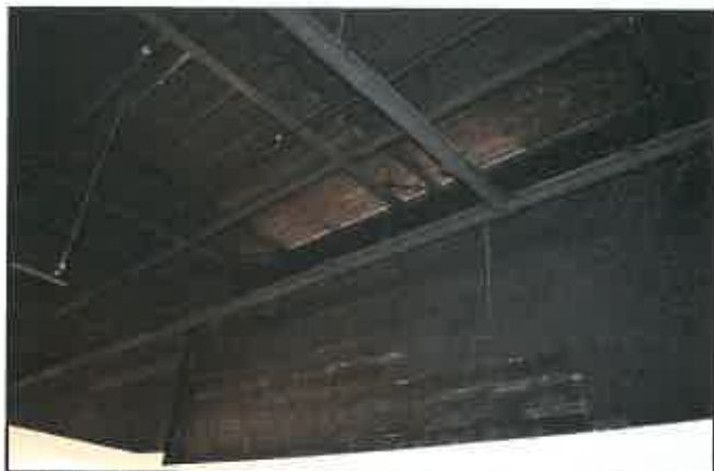
G. Item 3(Picture) Rust at roof deck
