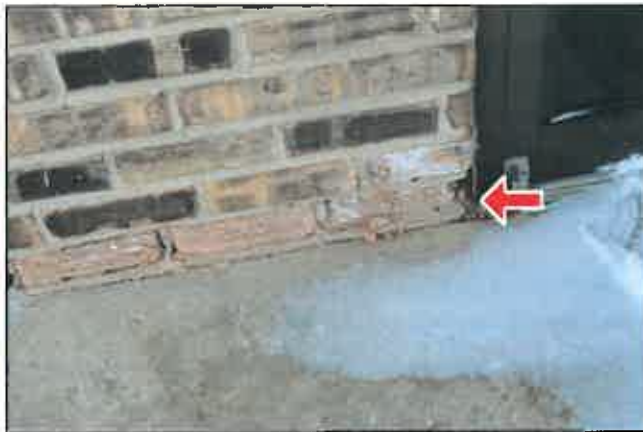
C. Item 2(Picture) Deteriorated bricks at entrance
