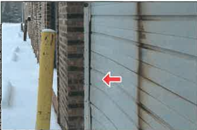
E. Item 10(Picture) Denting and misaligned door
