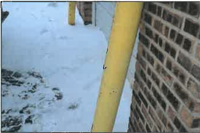
E. Item 9(Picture) Damaged bollard
