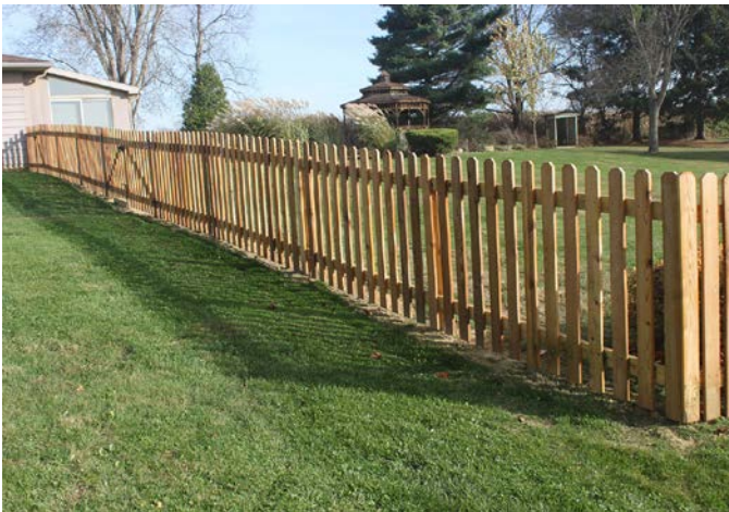
Left: Four-foot (4') high open design wood fence.
