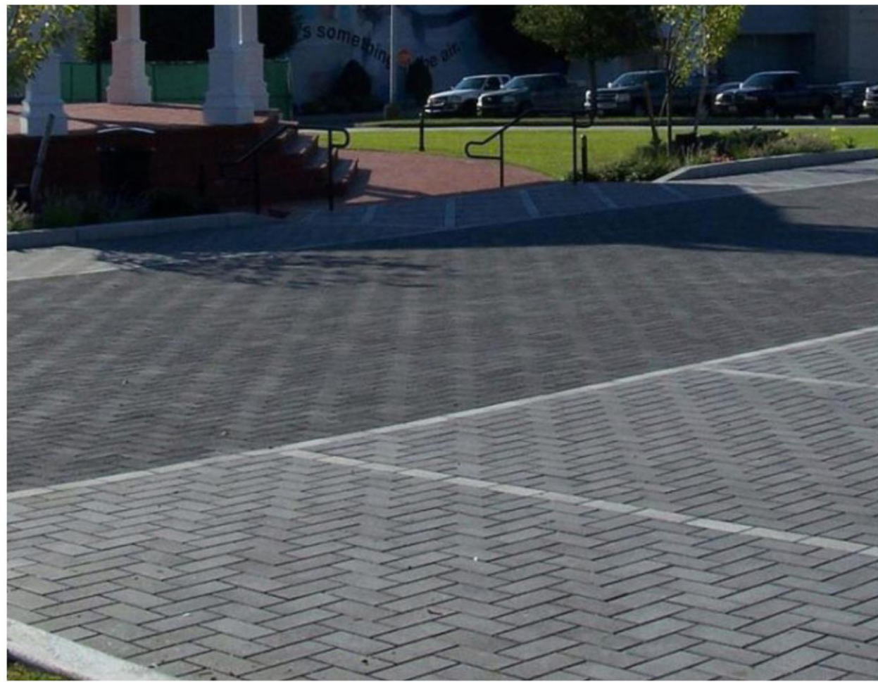
Permeable Paver Street - Unilock Eco Priora, 5"x10"
