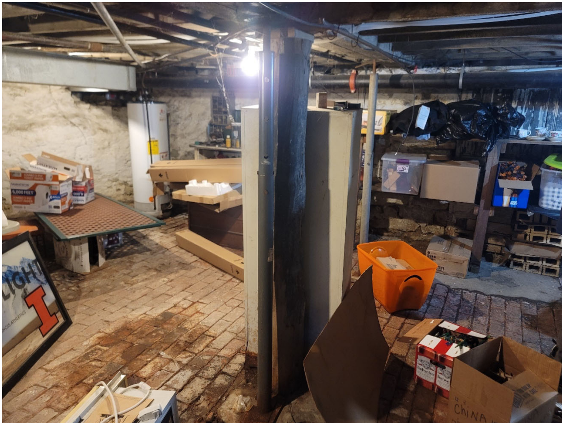
Figure 4 Wood column reinforcing first-floor framing
