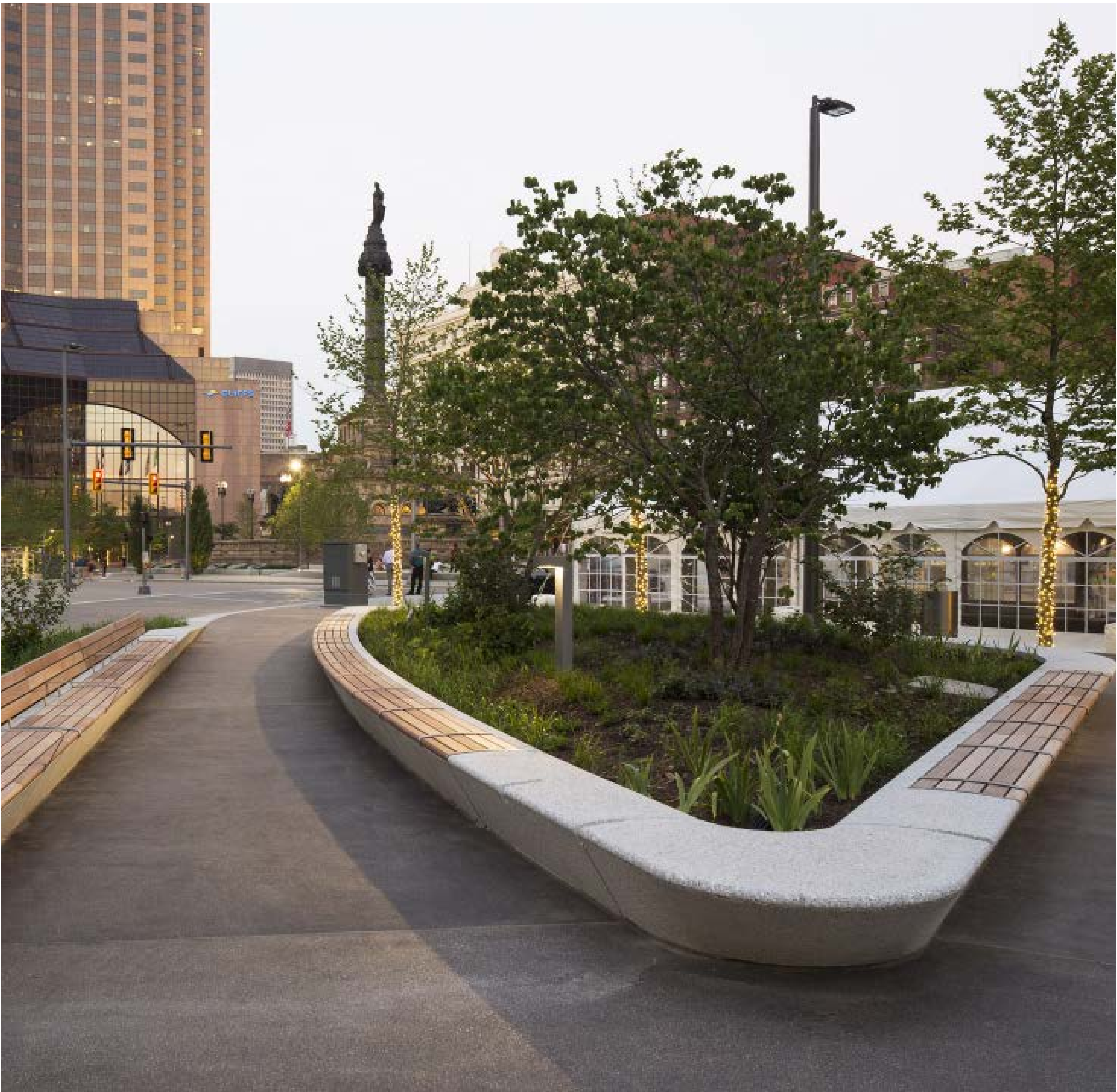
Poured-in-place concrete seatwall to have tapered profile.
