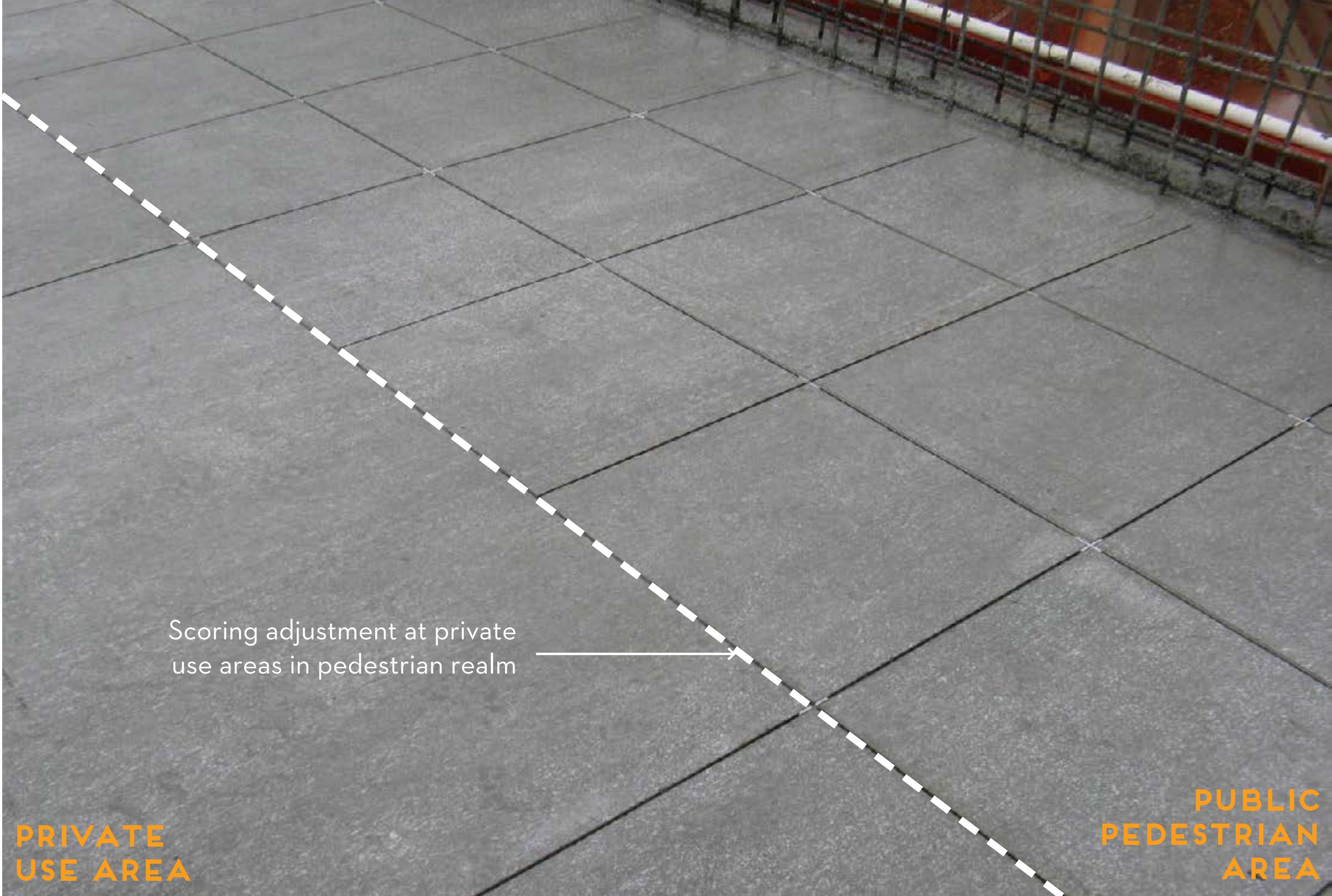
Scoring spacing to match the width of the sidewalk and be spaced no further than 6’ on center.
