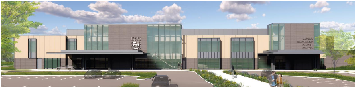
Final Proposal - This last image incorporates face brick on the base and the main entrances but in a gray stone. This brings the building closer to the masonry requirements with 38% face brick; 19% precast panels; 31% glass and 11% metal panels. A variation is still required.
