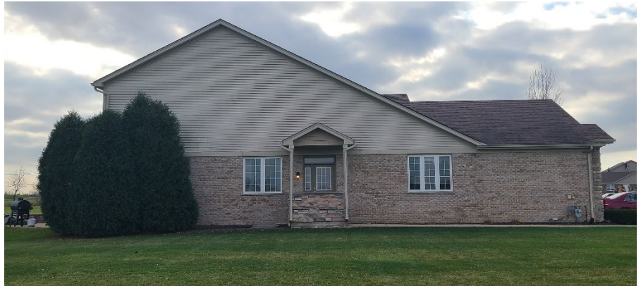
Existing side elevation: Expansive siding, Narrow door entry w/ downspouts & stone accent.
