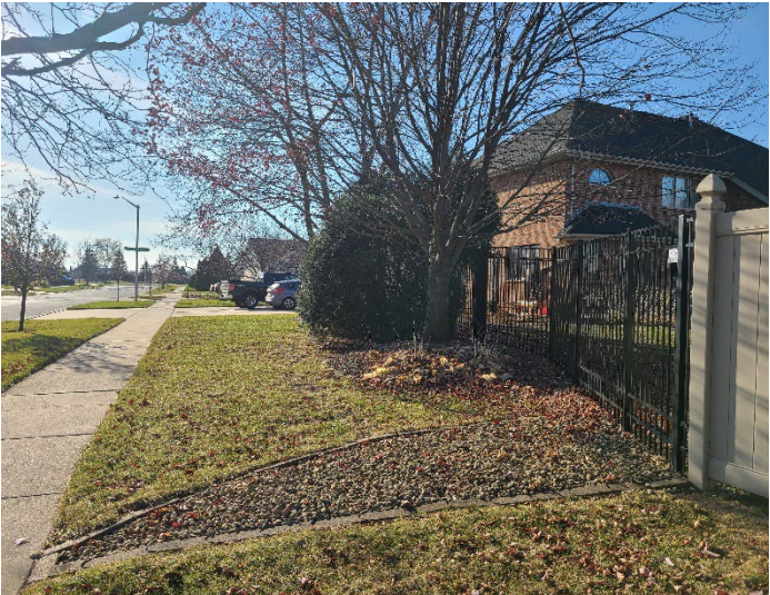
Installed fence, Noncompliant; 12'-7" to property line, angled jogging
