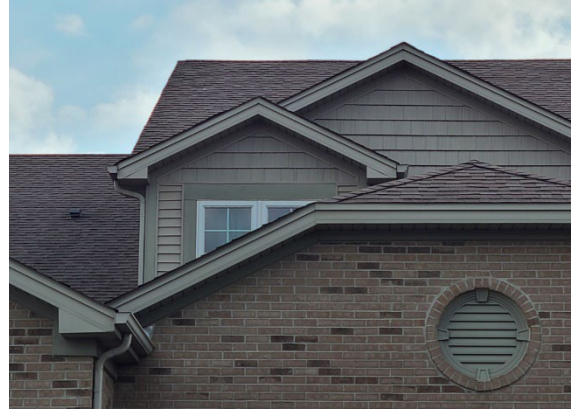
Existing detail in shingle variety and cedar trim
