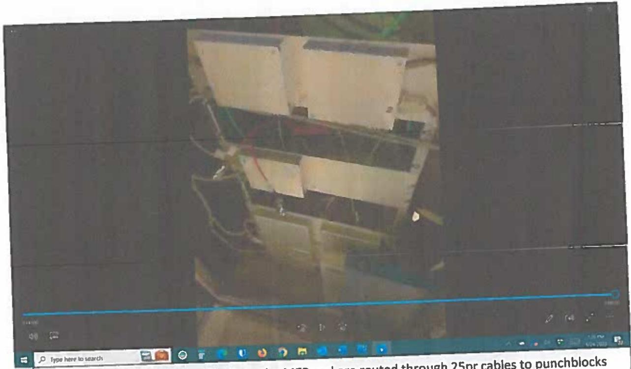
This photo shows the voter I/Os from the MEP and are routed through 25pr cables to punchblocks to be installed on data room wall above
