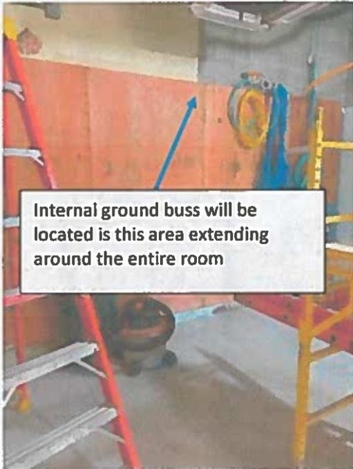
Internal ground buss will be located in this area extending around the entire room
