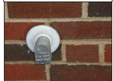
Sample Outside Vent for Indoor Gas Meter
