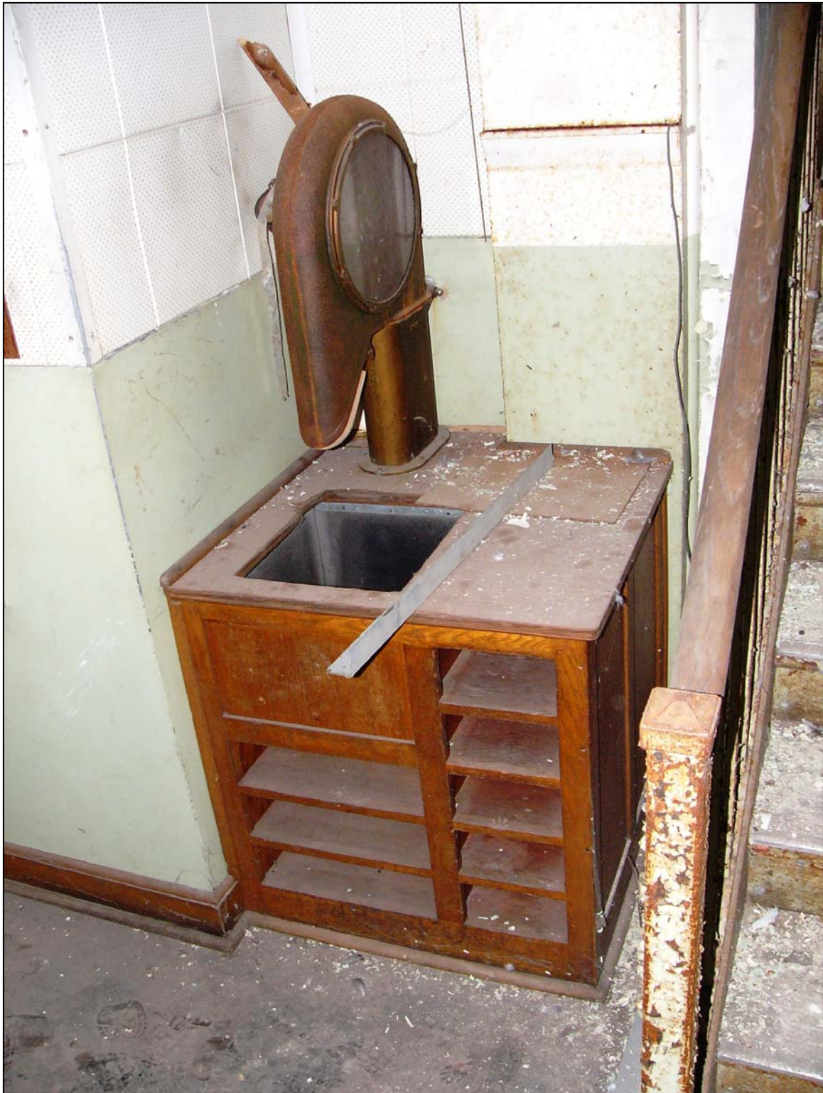
Second Floor, Building 48A. The remnants of a pneumatic tube conveyance system can still be found near the stairs to the second floor of Building 48. Photograph by J. Trnka, July 2005.
