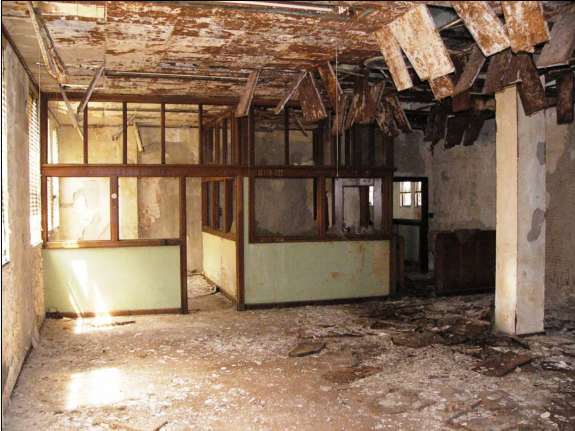
Second floor of Building 48, office area. As shown here, the leaking roof and compromised windows have lead to a significant amount of water damage, especially on the second floor. Ceiling tiles and wall plaster has been destroyed by water and the entire floor is generally covered by a layer of dust and bird waste. Photograph by J. Trnka, July 2005.
