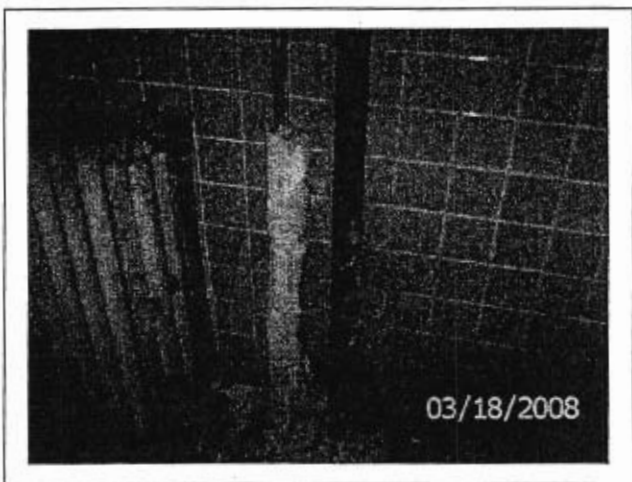
PHOTO 5 Viewing 2" pipe insulation, women's restroom. ACM Sample #48-08
