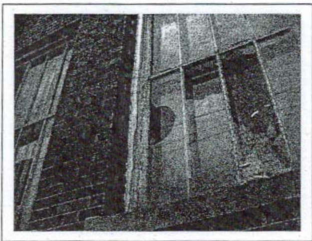
PHOTO 29 ACM Sample #48-59 Viewing asbestos-containing white window caulking, Exterior.
