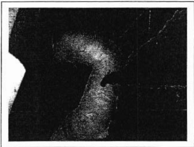
PHOTO 9 Viewing 10" pipe insulation, Basement near tunnel. ACM Sample # 48-20
