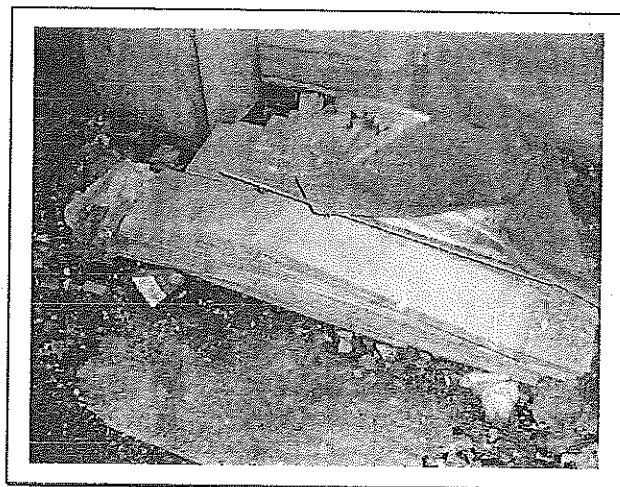
PHOTO 32 Viewing transite panels, 1 st floor North entrance. ACM PACM
