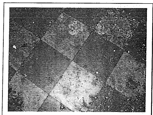
PHOTO 18 Viewing 9"x 9" VFT white and blue checkerboard pattern, 3 rd floor – North central room. ACM Sample #48-19
