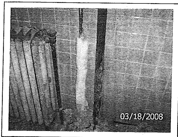
PHOTO 5 Viewing 2" pipe insulation, women's restroom. ACM Sample #48-08
