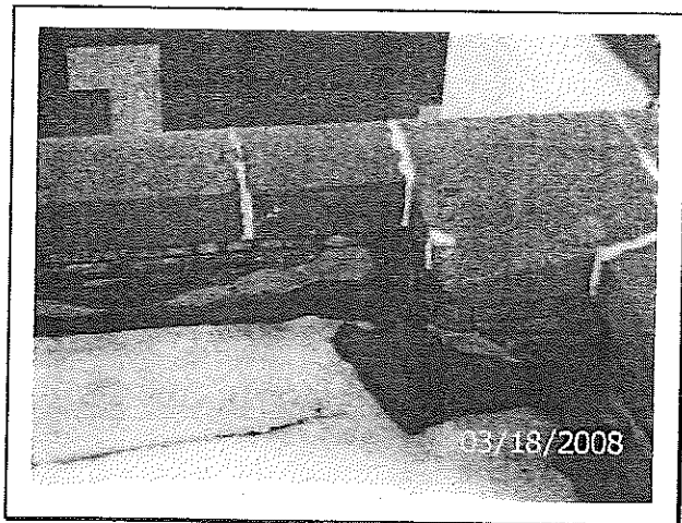
PHOTO 27 Viewing asbestos-containing roof flashing, Throughout roof. ACM Sample #02A
