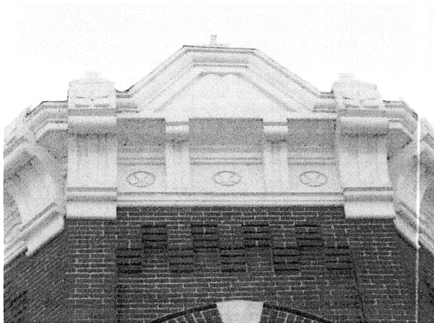
Figure 2 Detail of metal cornice atop the canted corner. Photo by Tallgrass Historians L.C., 2008
