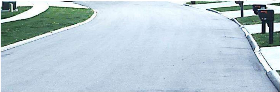
Figure 11: Example of “Very Good” Condition (HMA) – Mourning Dove Dr This picture was taken from the 2018 data collection records. Mourning Dove Drive, north of Hummingbird Circle has a nearly perfect PCI of 97/100 because it demonstrates no visible pavement distresses.
