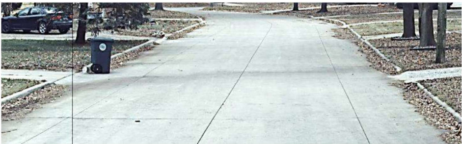
Figure 12: Example of “Very Good” Condition (PCC) – Seneca Ave This image shows Seneca Avenue from the 2018 data collection, in which it was rated as 86/100 and would be considered “Very Good” for a PCC pavement.
