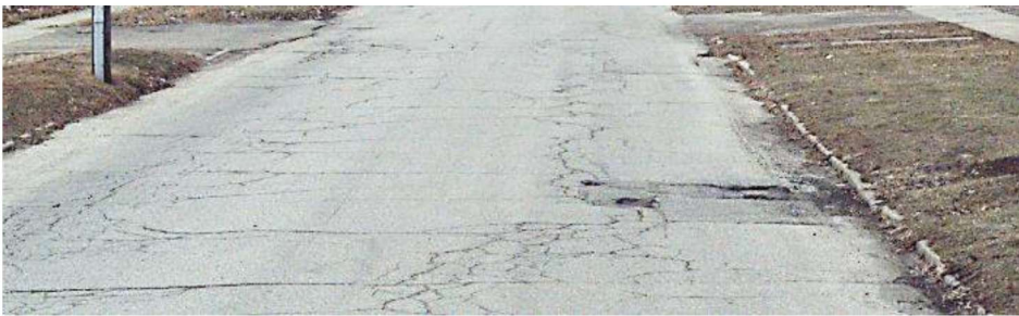
Figure 17: Example of “Poor” Condition (HMA) – Sumner St This image shows an HMA street whose pavement is rated as 33/100 and considered to be in “Poor” condition. Sumner Street, east of 4th suffers from widespread cracking and a few points of more severe failure that may likely cause impacts to drivers.
