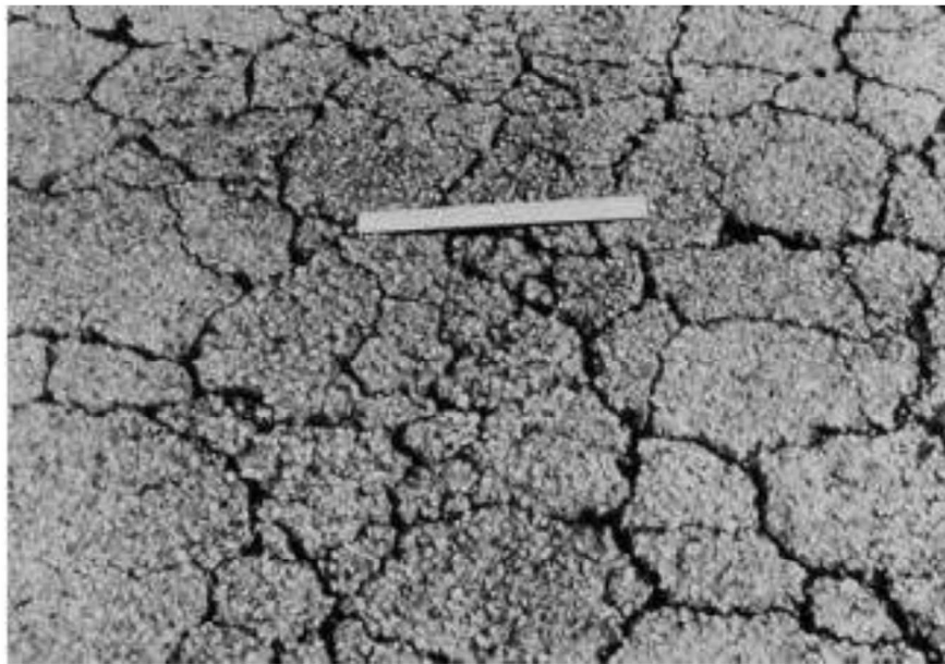
Figure 4: Example of Alligator Cracking (ASTM) This image is from the ASTM D6433 “Standard Practice for Roads and Parking Lots Pavement Condition Index Surveys.” Alligator Cracks are when pavement breaks into a “scaly” pattern typically caused by fatigue, either from repeated heavy loads, lack of sufficient subgrade support, or weakened material due to drainage issues.
