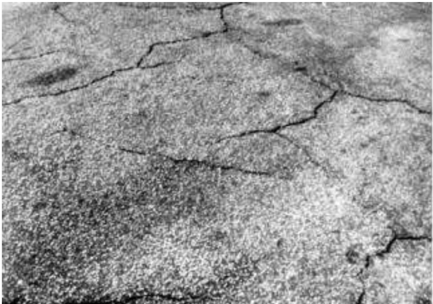
Figure 5: Example of Block Cracking (ASTM) This image is from the ASTM D6433 “Standard Practice for Roads and Parking Lots Pavement Condition Index Surveys.” Block cracks are when pavement breaks into “chunks” or “blocks” that are roughly rectangular, caused by internal stress from temperature or lack of lateral support.
