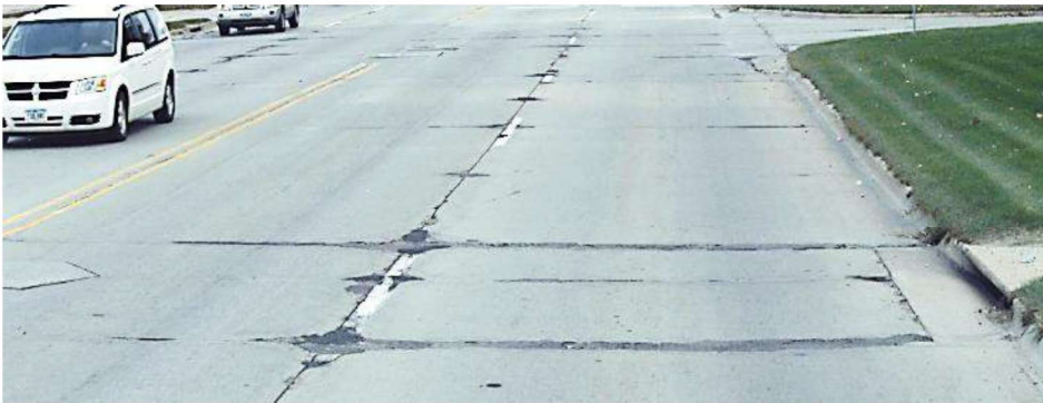
Figure 16: Example of “Fair” Condition (PCC) – Ansborough Ave This picture of Ansborough Ave between Stratford and Upton is an example of a PCC pavement that was rated as 51/100 which would be considered “Fair.”
