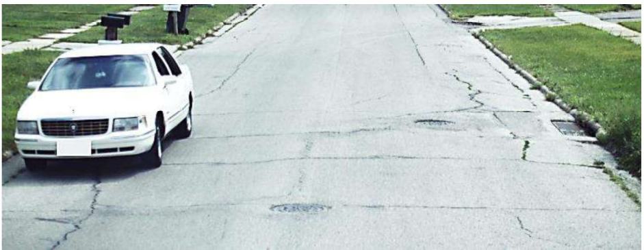
Figure 15: Example of “Fair” Condition (HMA) – Oleson Road This image of Oleson Road between Hammond and Bethel is an example of HMA pavement in “Fair” condition, with a PCI of 48/100. There are very noticeable distresses but they only impact drivers slightly.
