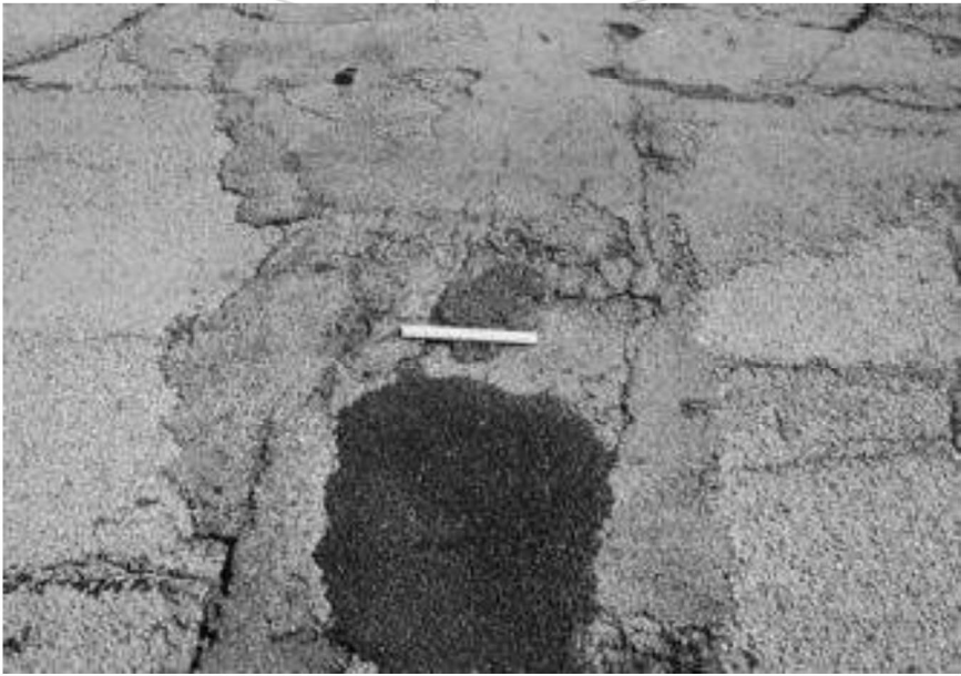
Figure 8: Example of Patching (ASTM) This image is from the ASTM D6433 “Standard Practice for Roads and Parking Lots Pavement Condition Index Surveys.” Patching is the result of corrective actions already taken and are indicative of underlying issues as well as a common point of failure.
