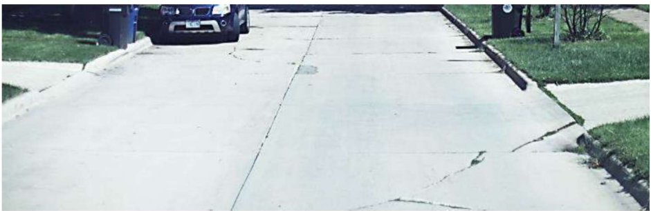
Figure 14: Example of “Good” Condition (PCC) – Kingsley Ave This image shows an example of a PCC pavement in “Good” condition. Kingsley Avenue between Fletcher and Lawnhill is rated as 69/100, because of a few cracked panels and small patches in decent repair.
