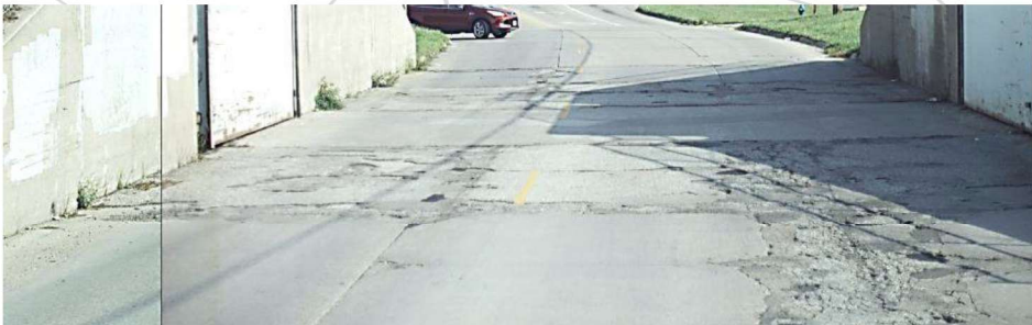
Figure 21: Example of “Very Poor” Condition (PCC) – Fletcher Ave This picture of Fletcher Street south of Black Hawk Road is the only PCC pavement of “Very Poor” condition in Waterloo. Rated as an 8/100 in 2018, it exhibits multiple points of severe distress that could not be addressed through any means other than rebuilding the road from the base up.
