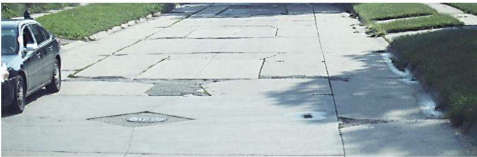
Figure 18: Example of “Poor” Condition (PCC) – Webster St This image is an example of a PCC pavement in “Poor” condition. Webster street between Linn and North Barclay was rated as 26/100 due to uneven joints and numerous point failures that would certainly impact driver experience.
