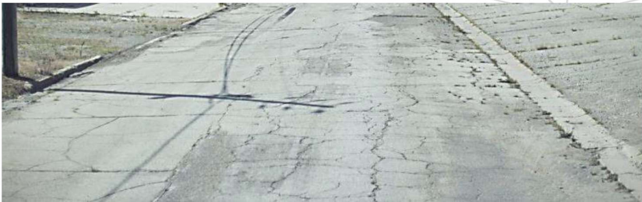
Figure 19: Example of “Very Poor” Condition (HMA) – 10 th St East This picture of 10 th Street East, to the southwest of Sycamore street is one of the few HMA pavements in Waterloo considered to be in “Very Poor” condition. Rated as 17/100, this road’s pavement exhibits distresses across the entirety of the street and even has grass growing through the cracks.
