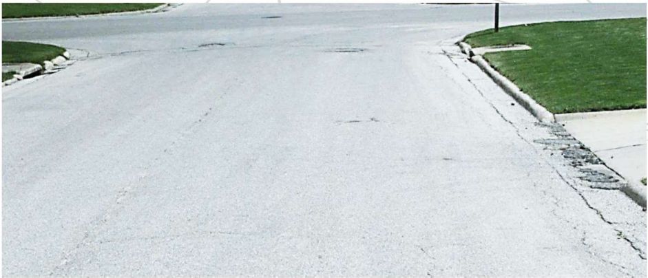
Figure 13: Example of “Good” Condition (HMA) – Liberty Ave This picture of Liberty Ave between Oregon and Minnesota. It was rated as 75/100, which would be considered good for an HMA pavement. Low severity cracks and small distortions can be found, but nothing that impacts drivers.
