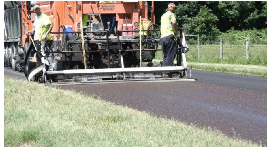
Figure 30: Microsurfacing Crew at Work (Eric Pulley). This is picture shows a crew using a Microsurfacing machine to lay a new surface on this street.
