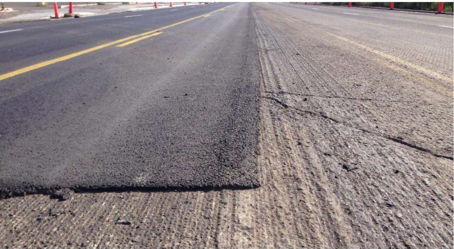
Figure 27: HMA Overlay Placed On Milled Pavement (Famartin) This is a picture of an asphalt overlay placed on I-80 through Elko, Nevada after part of the original pavement was milled off.
