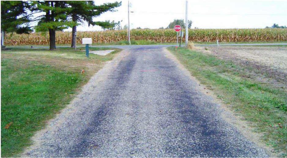
Figure 37: Rural Chip Seal Road (Ben Grimm) This is an example of typical chip seal road. This road near Kempton Indiana exhibits raveling, bleeding, and weathered aggregate indicative of an older pavement in need of a new coat
