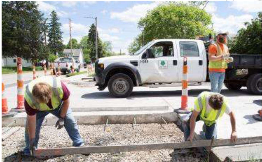
Figure 32: PCC Restoration (City of Cedar Rapids). This is a picture of a city maintenance crew in Cedar Rapids performing a panel replacement as part of a larger concrete restoration project.
