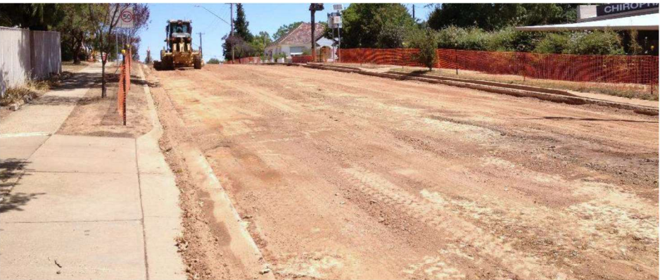
Figure 26: Reconstruction of Micheltmore Street (Bidgee) This photo shows a road torn out and being prepared for reconstruction
