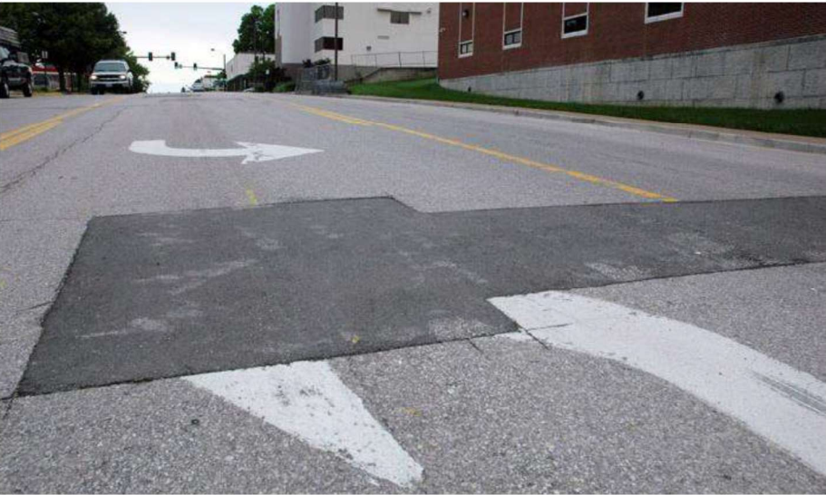
Figure 36: HMA Patching with Localized Pavement Removal (KOMU) This is an example of an asphalt patch applied with appropriate localized removals and some base repair.
