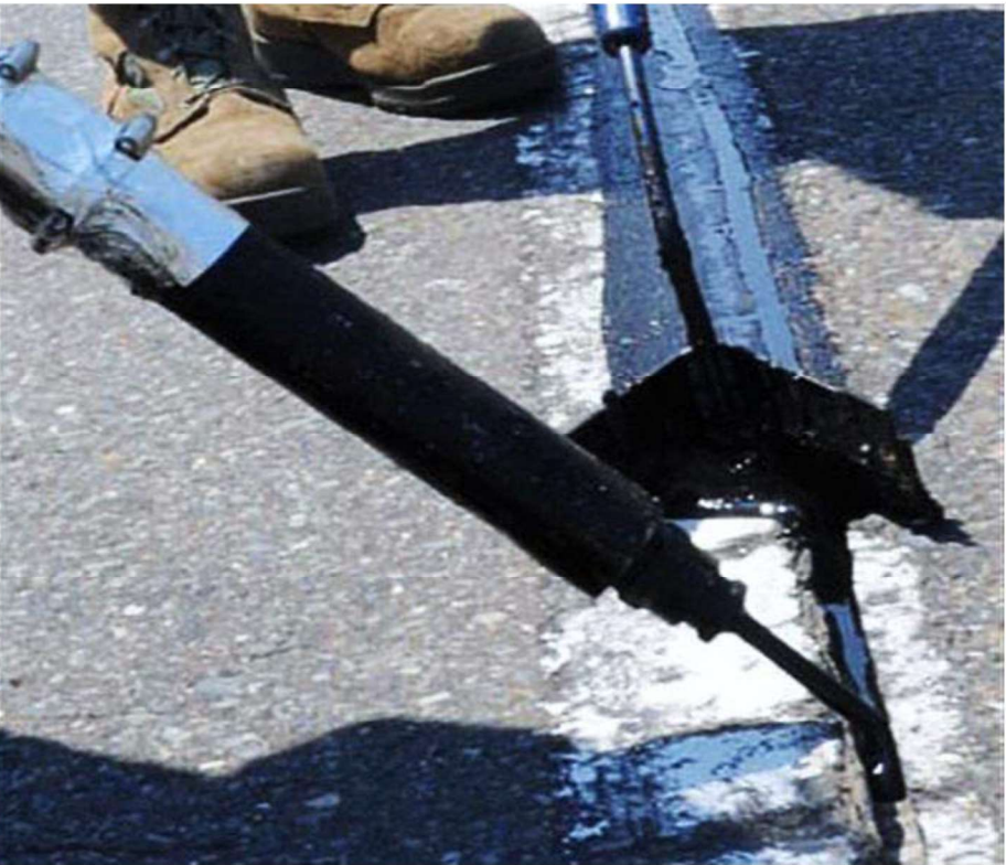
Figure 35: Crack Sealing Performed W/ Routing (USAF/Kenna Jackson) This is an example of crack sealing being performed with special preparation in the form of using a router to clean up the crack profile, as being performed by 35th Civil Engineer Squadron.
