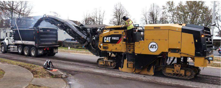
Figure 28: Cold Milling Machine (Anthony Neff) Cold Milling Machines like the Caterpillar PM 622 above are used to strip off the top layer of pavement. Those millings could then be used for in-place recycling, or the pavement could receive a new 3” overlay.
