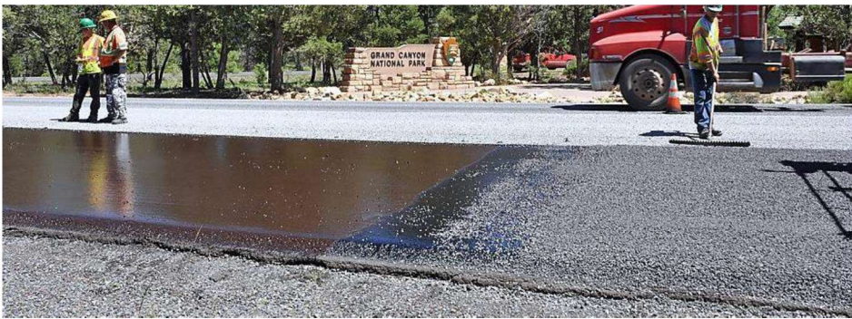
Figure 34: Cape Seal (Michael Quinn-NPS) This picture taken by the National Parks Service near the entrance to Grand Canyon National Park shows a loose chip seal (right) that is having a slurry seal applied (left) to effectively turn it into a cape seal.
