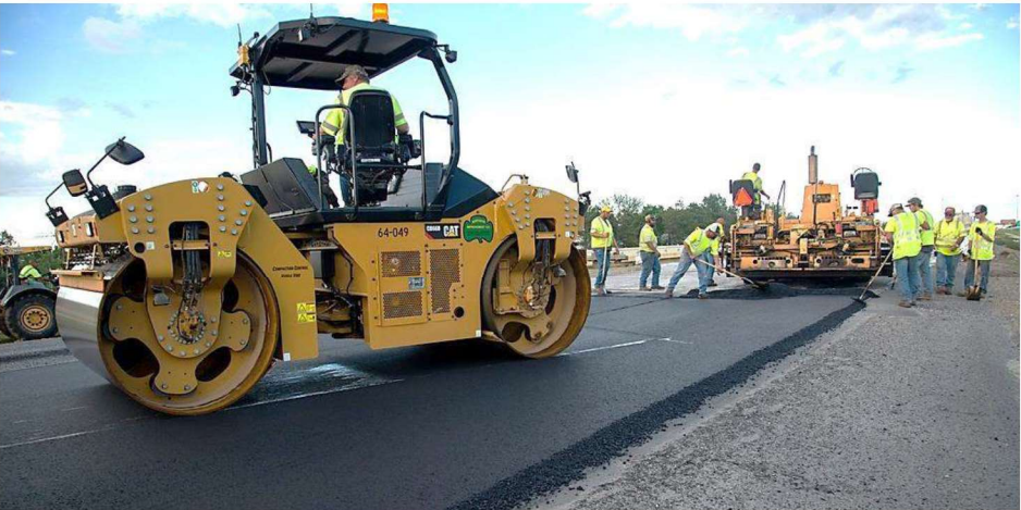
Figure 25: Reconstruction of I-94 (NDDOT) This photo shows the Construction of a brand new asphalt cement concrete pavement
