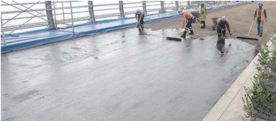
Figure 29: Slurry Seal Being Placed by Hand (Miraflores) This slurry seal is being placed to refresh the surface of the Villeno Rey Bridge in Miraflores, Peru.
