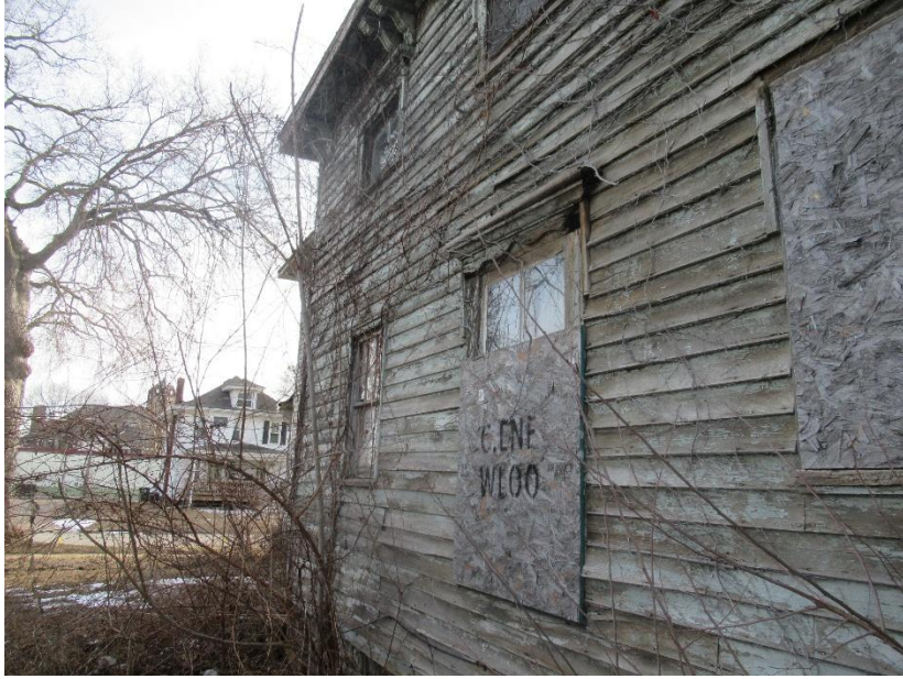
(East side of the building)
