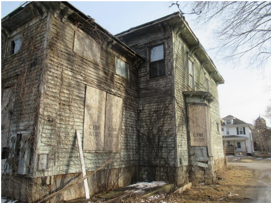
(East side of the house, looking from the rear)
