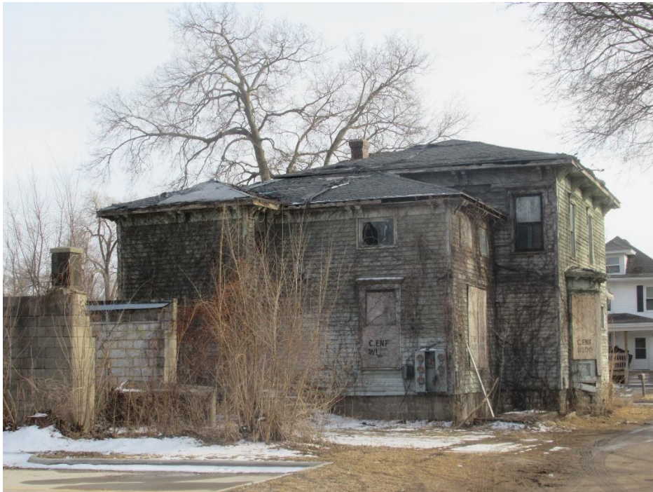
(Rear of the house)
