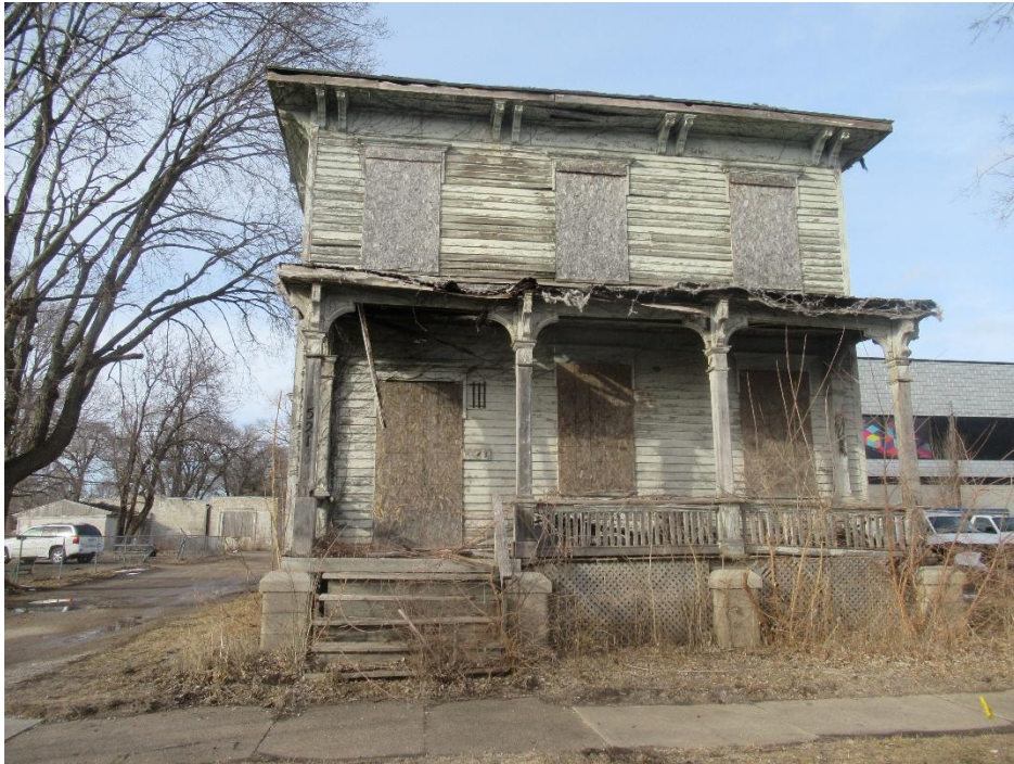
(The front of 521 Pine St)
