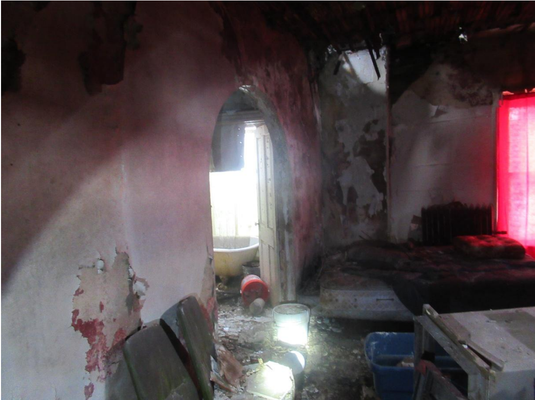
Interior photos 521 Pine Street- June 9, 2025
