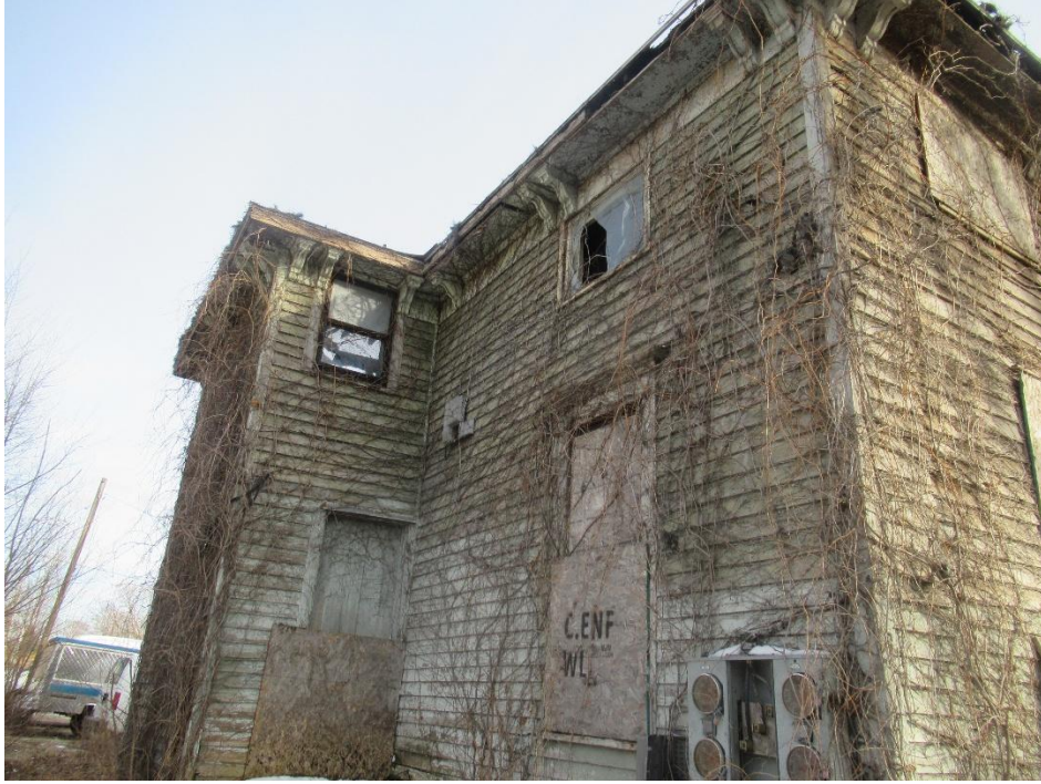
(Rear of the house)
