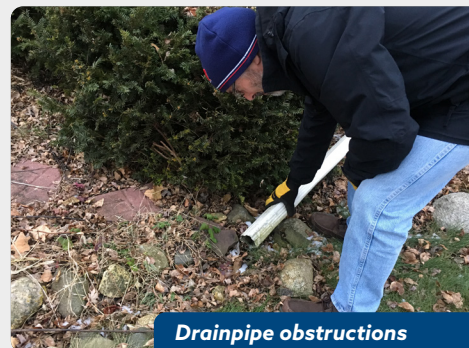
Removing sediment buildup
