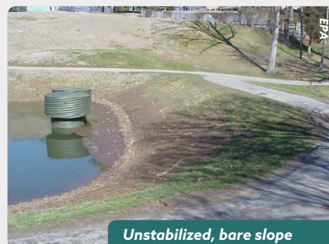
Clogged stormwater outlet
