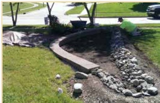
Rain garden under construction.
