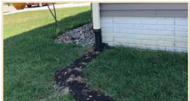
Buried drain pipe connected to downspout that discharges to the surface of a garden.
