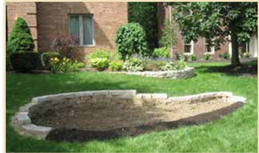
Upslope retaining wall around an oblong rain garden with a mulch berm on the downslope side.
