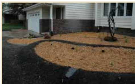
Rain garden berms under construction.
