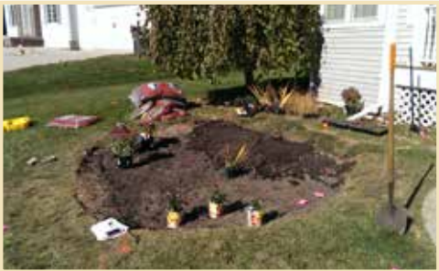
This rain garden was built below the yard surface with no berms. The water overflows onto the existing grass and flows away from the house.
