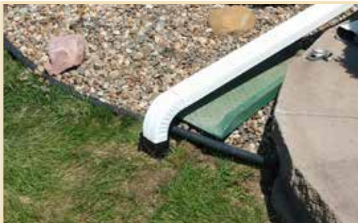
This rain garden is online with downspouts connected to underground drain pipe.
