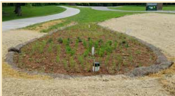
Enhanced rain garden with a vertical overflow structure.
