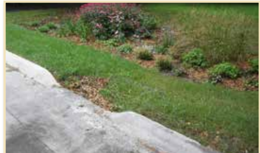
Pre-treatment grass filter strip used for a rain garden receiving street runoff.
