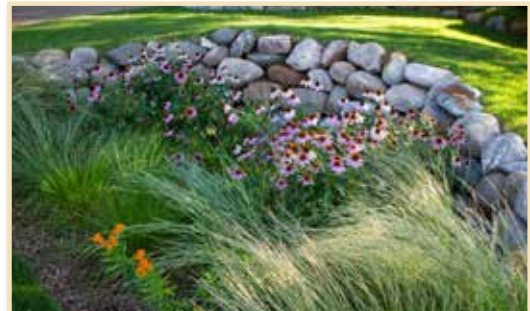
Rock retaining wall is cut into the slope to create a level bottom.
