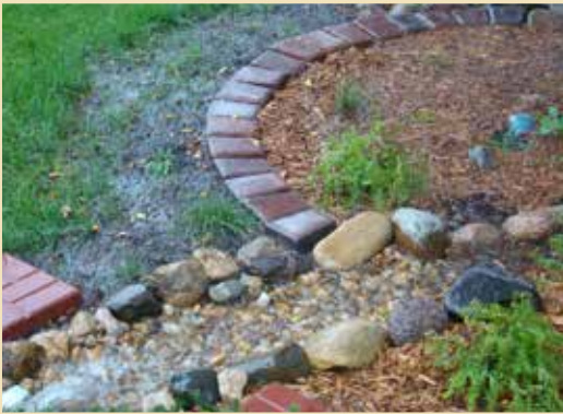
Rainwater enters the rain garden through a rock channel.
