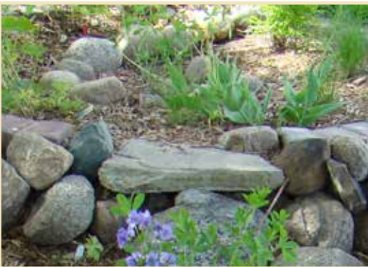
An outlet from a rain garden reinforced with rock.
