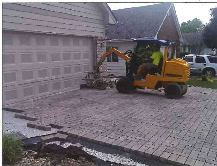
Step 4 Laying pavers
