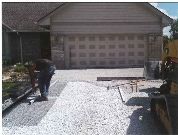
Step 3 Leveling and compacting aggregate
