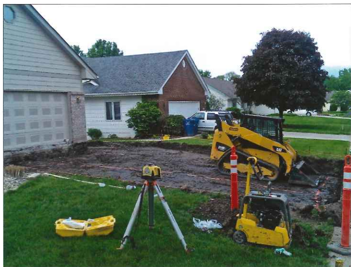
Step 1 Removal of concrete and excavation
