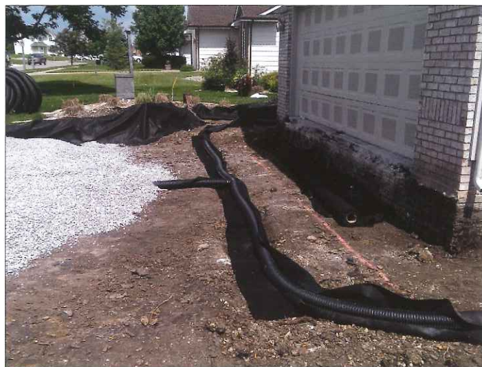
Step 2 Installation of perforated subdrain tile
