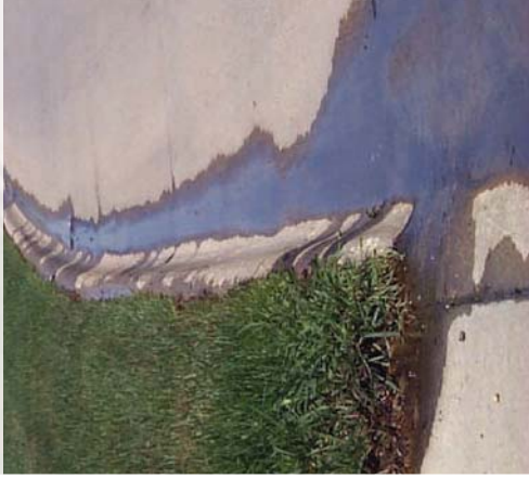
Water that should infiltrate is oozing off compacted turf and into the storm drain.
