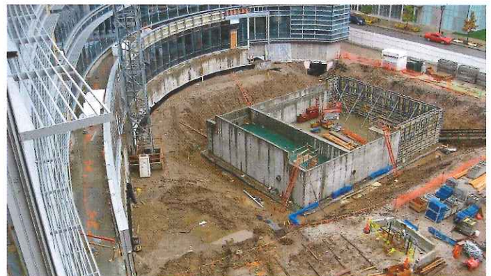
The Wellmark Building in Des Moines constructed this large cistern. The water is collected for irrigation, and supplies 8,000 gallons a day for flushing urinals and toilets. It reduced Wellmark's treated drinking water use by nearly 58%.
