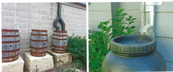
Left: Connected rain barrels capture more water for reuse. Right: A downspout is redirected into a rain barrel.
