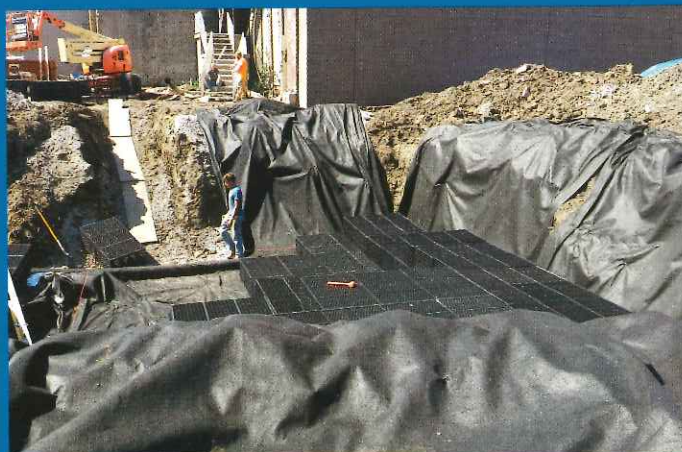
These structural blocks and plastic liner are used to store water below ground. They are used as the reservoir below natural or landscaped water features, like shown above and on the front page.
