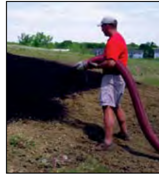
Compost being spread over the soil prior to seeding or sodding.
