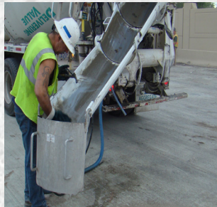
SELF-CONTAINED CHUTE WASHOUT
