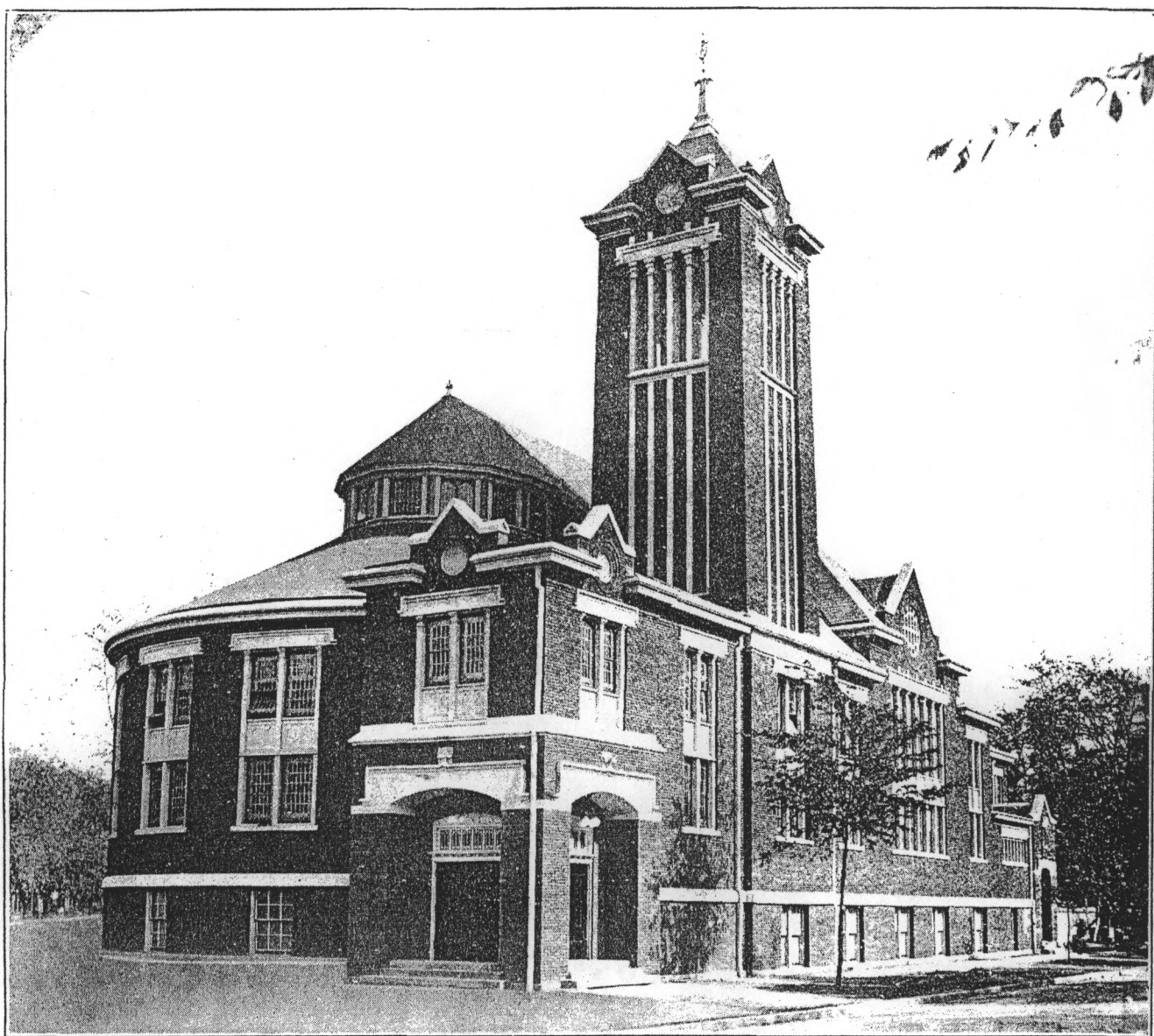
SECOND BUILDING WALNUT STREET BAPTIST CHURCH, ERECTED 1908 CLINTON SHOCKLEY, ARCHITECT CHARLES WASSON, BUILDER
