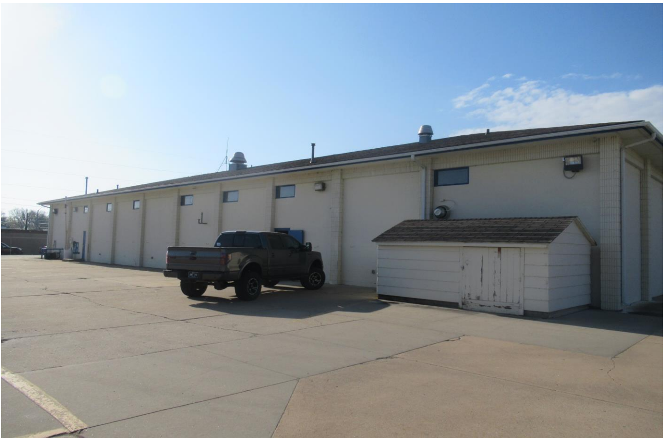
Picture 5: Rear of the existing building.
