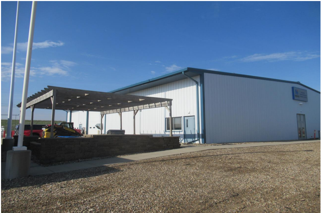
Picture 1: Existing Hawkeye RTTC building.
