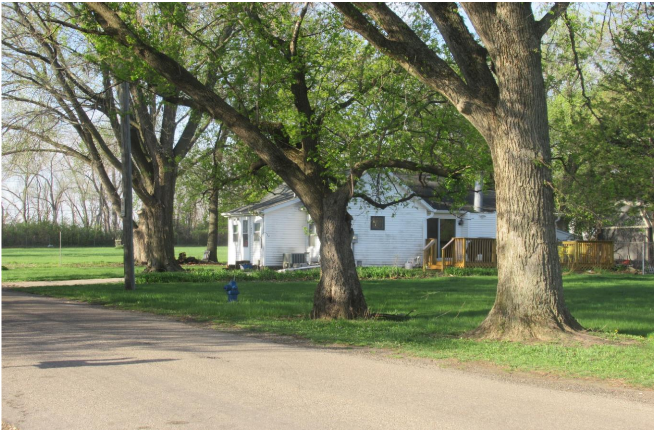
Picture 7: Looking at 1925 Avon Avenue.
