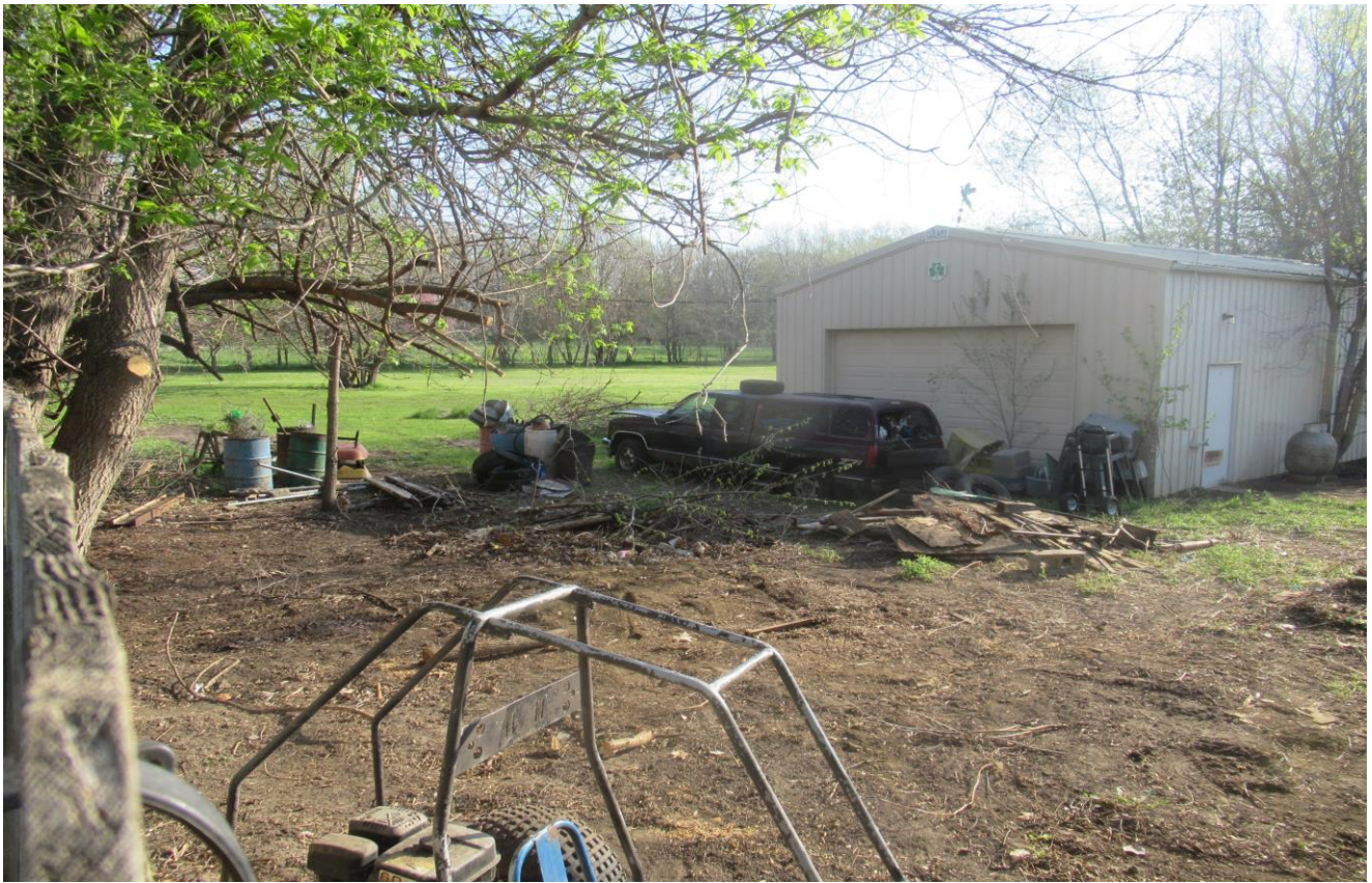
Picture 3: Looking at second accessory structure.
