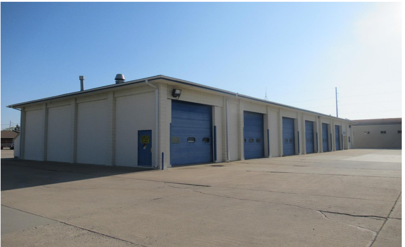
Picture 1: Existing Building
