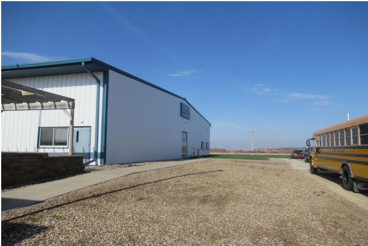
Picture 5: North side of the building.
