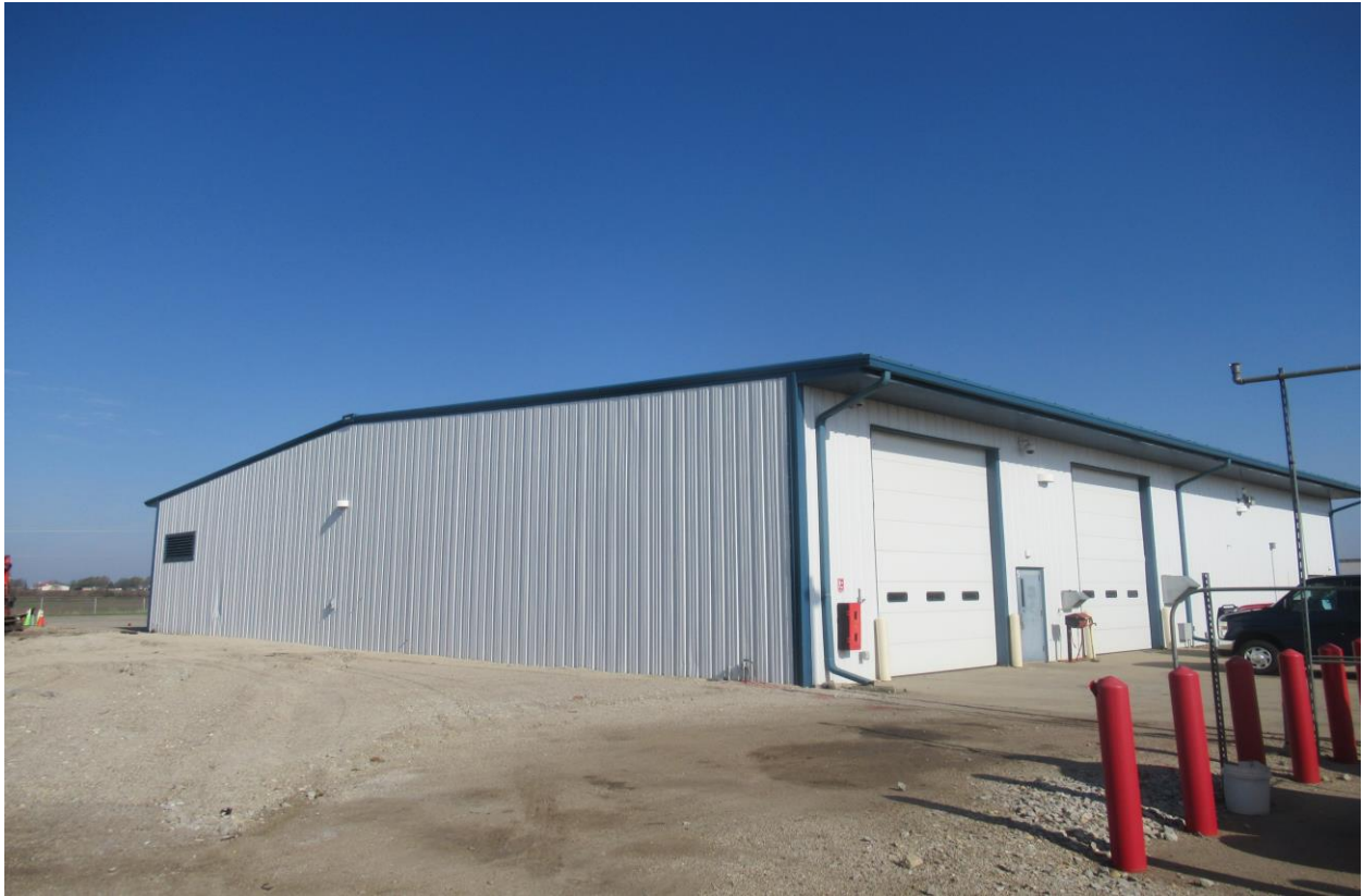
Picture 3: South side of existing RTTC building.
