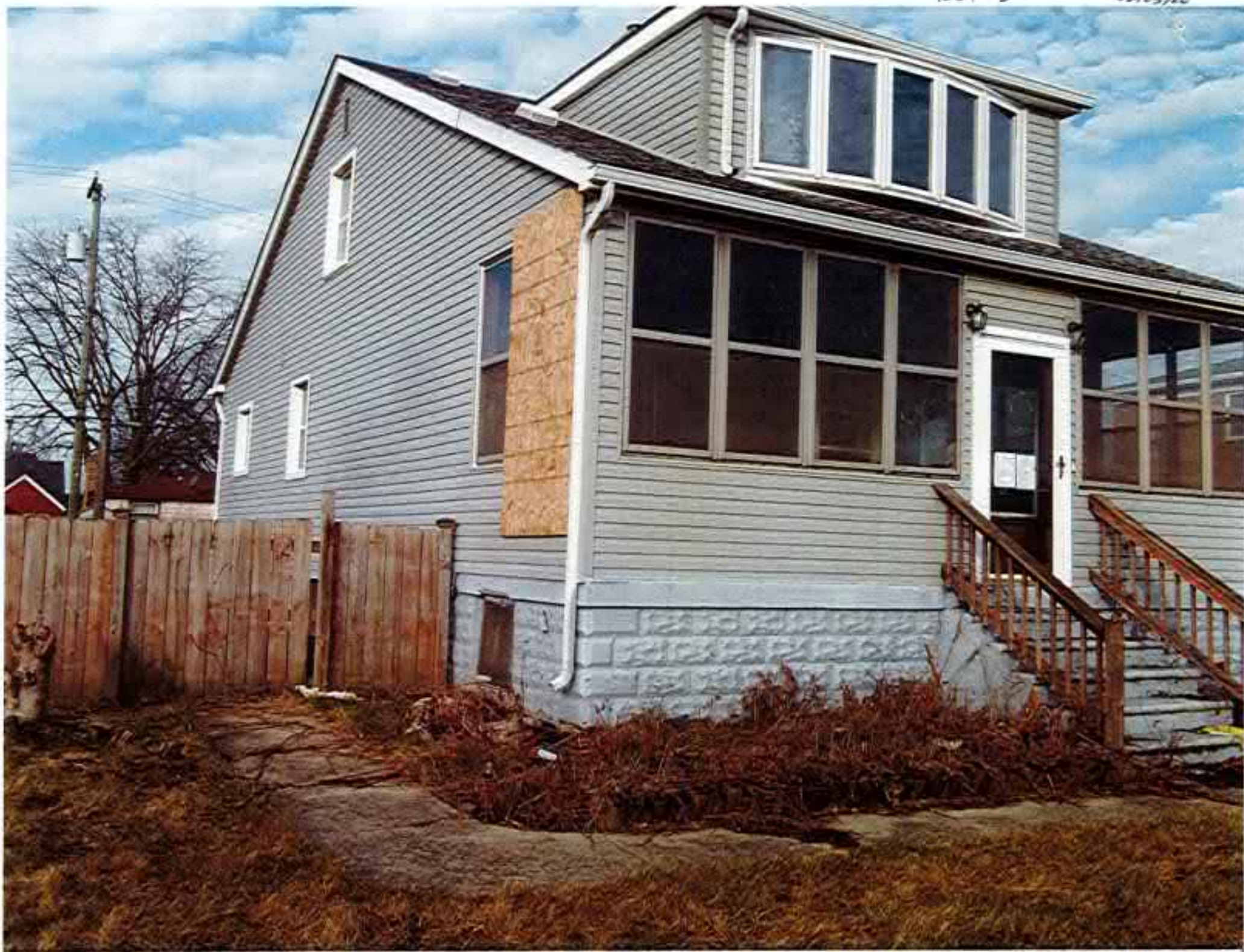
NDS REMAINS SUBSTANTIAL DAMAGE WITH 2 SEVERE MISSING FRONT WINDOW (P)
