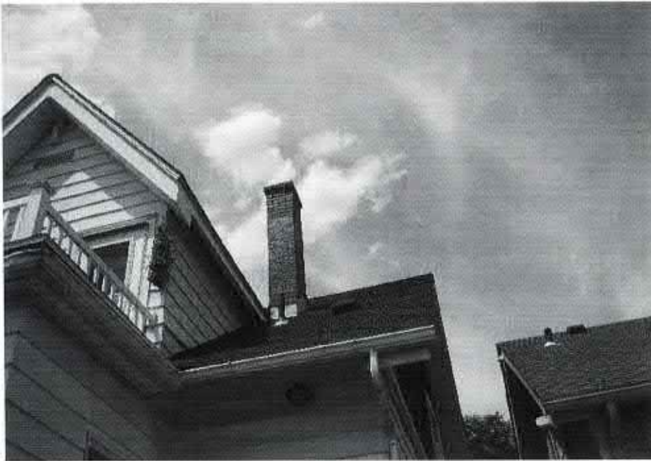
CHIMNEY NOTE: NO OPEN MORTAR JOINTS.
