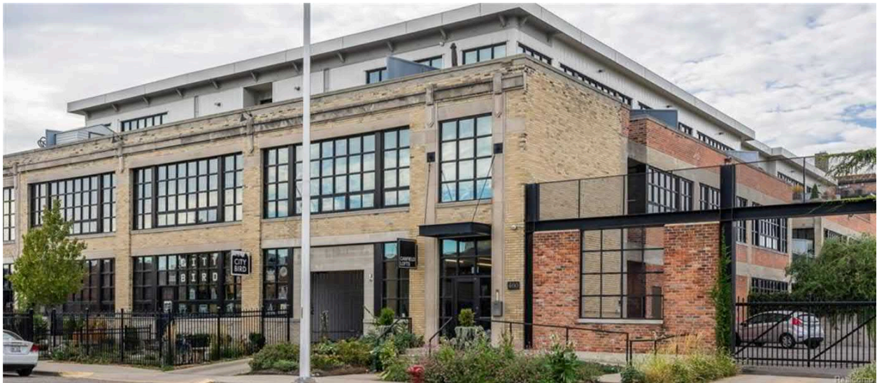
As a conceptual example, pictured here is 460 W Canfield in Detroit, an existing 2 story masonry structure with a 3rd story added, and retail facing the main street.
