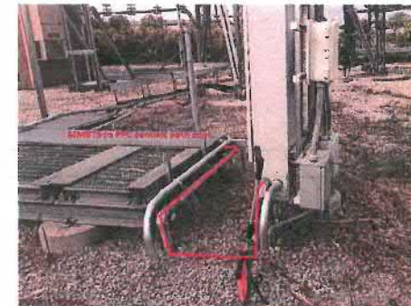
ENTIRE CONDUIT PATH FROM PPC TO MMBTS
