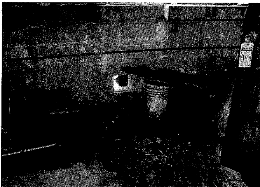
Site: Detroit Tubular Rivet Photograph No.: 26 Direction: West Subject: Hole in the wall of the Detroit Tubular Rivet facility and evidence of animal access
